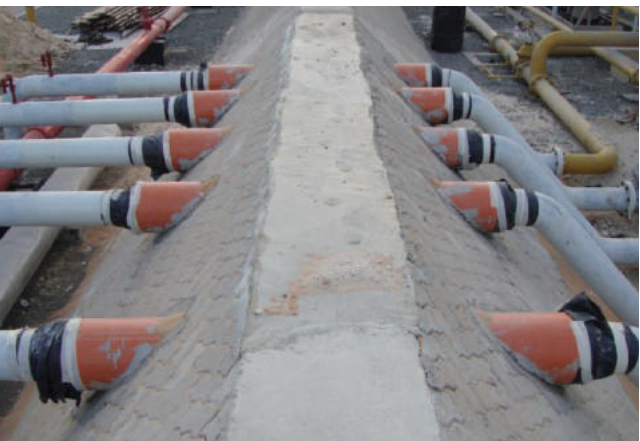
Site Execution - Piping
