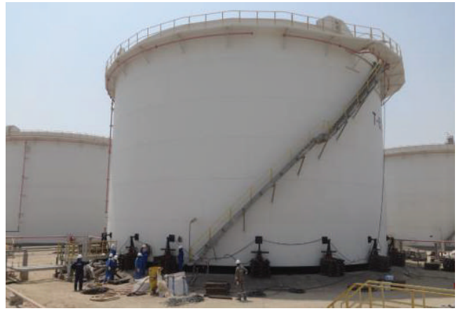
Jacking System - Storage Tanks
