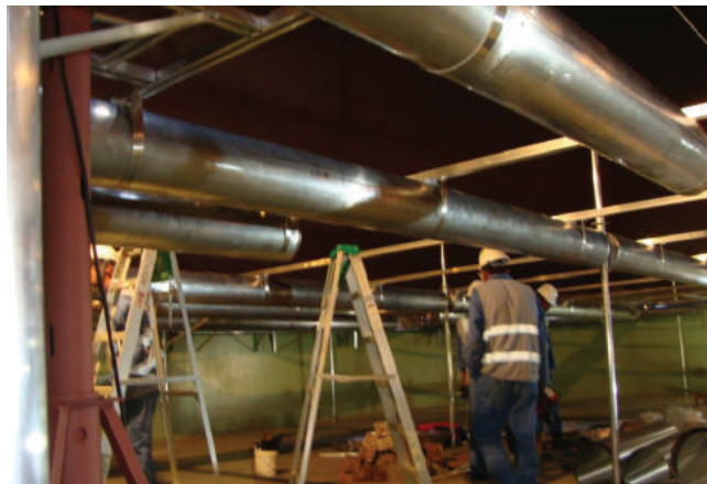
LRUT Inspection of Underground Piping
