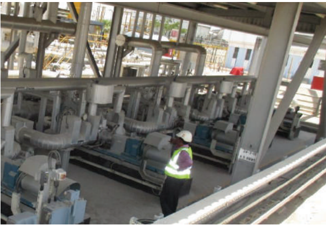
Pump House Inspection
