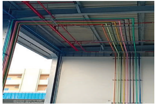
Utility Piping Installation
