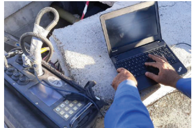
Inspection of Equipment MEP
