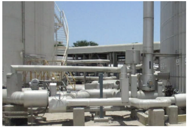
Tankfarm Cladding & Insulation
