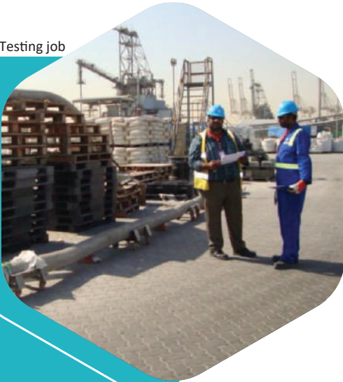
Pump Inspection & Maintenance
