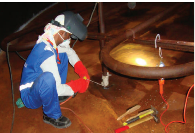
Tank Confined Space Works
