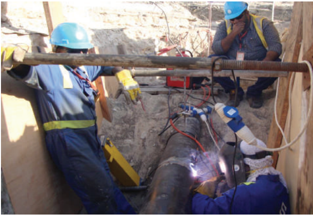
Underground Piping work
