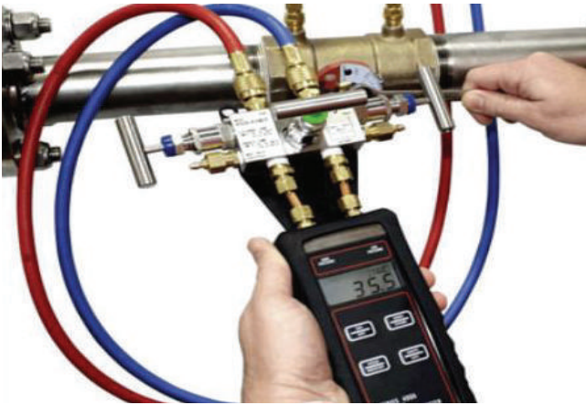
Air Conditioner Work MEP
